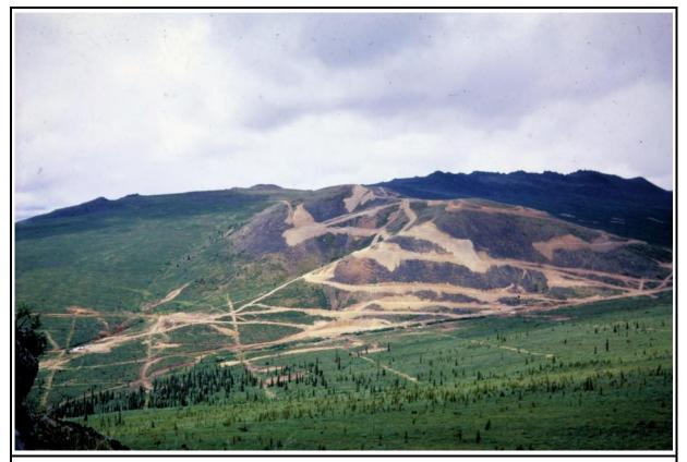
*Figure 1. Looking north to Patton Hill at the Casino calcalkaline copper-gold-molybdenum porphyry deposit in central Yukon, Canada. The deposit is related to a calcalkalic stock. 1971 photo, looking northwest, shows the rusty limonite thumbprint and large size common to porphyry deposits.*
